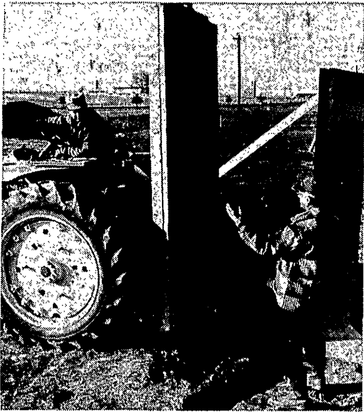
Concrete sandwich wall panel is set in a notched foundation. Threaded rods will be installed to anchor each panel to the building floor. This self-anchoring design, developed by University of Illinois agricultural engineers, eliminates need for supporting columns to hold walls in place.
