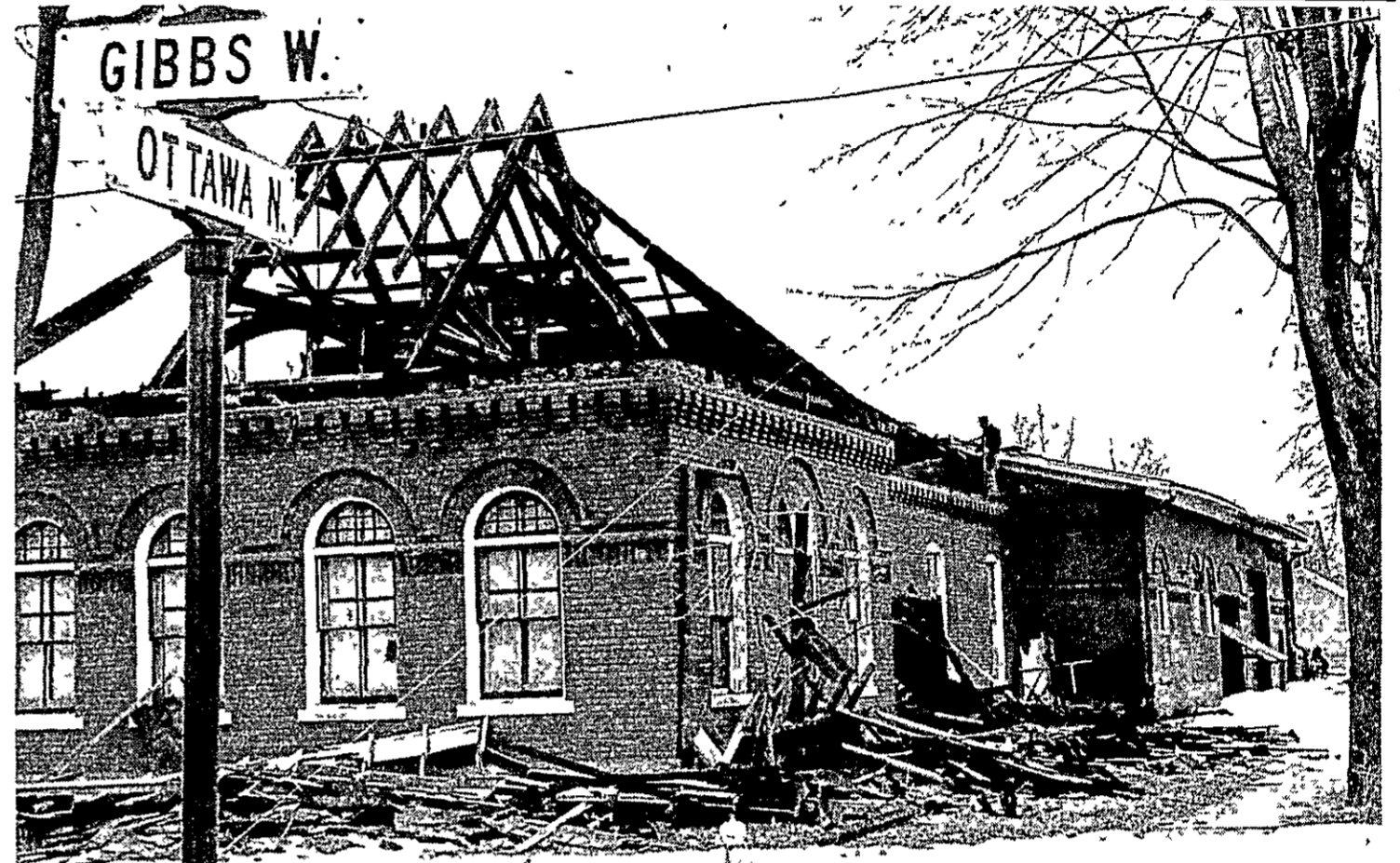
OLD CITY DPW GARAGE, WATER PLANT COMING DOWN
