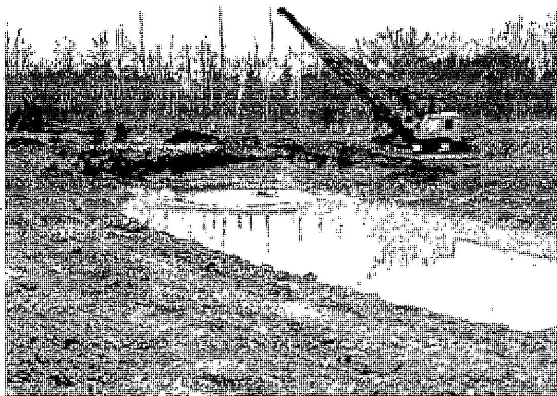
A farm pond is being constructed on the farm of C.W. Durst in Eagle Township. The contractor is Ed. Mathews. The Durst pond will be 200 by 80 feet in size.
