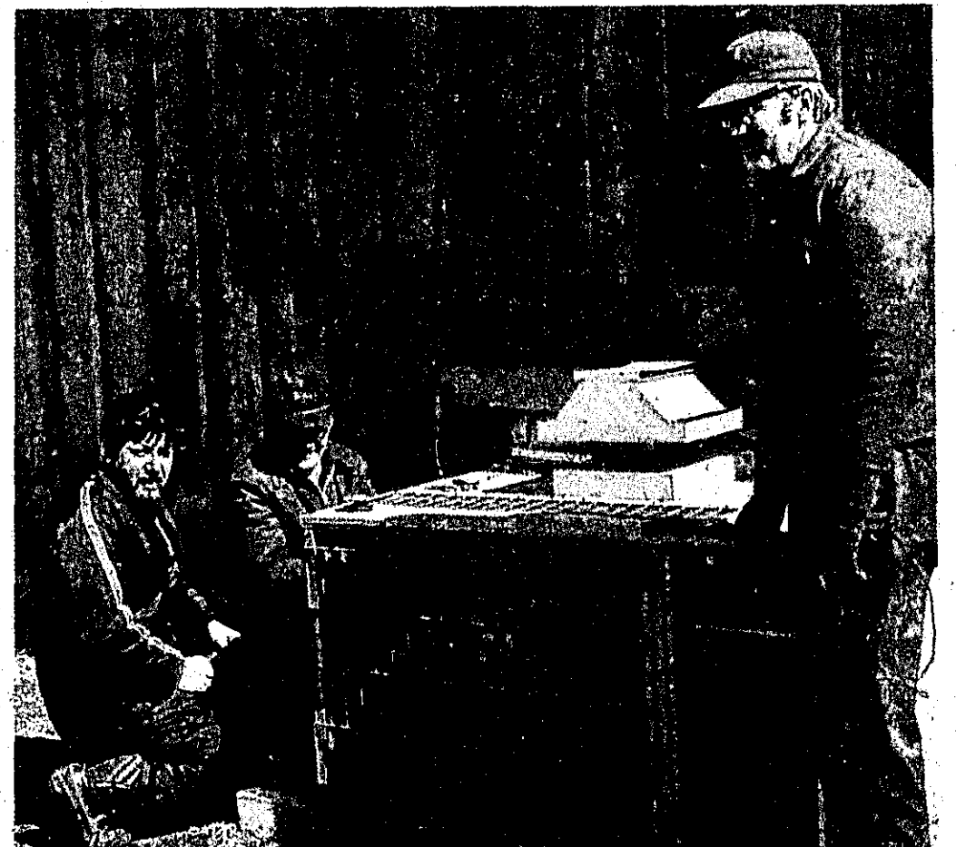
John [Jack] MacLennan from Rainbow Lake, Larry Schafer of Fowler and Joe Ondrus of Middleton working on a portable generator for the furnace in Dr. Steigerwald's office in Maple Rapids. Generators were in high demand when power sources gave out throughout the county.
