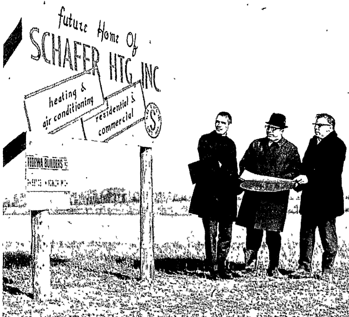
Groundbreaking for a new 40x100-foot home for Schaffer Heating Inc., will be sometime this month at the firm's new location five miles south of Fowler. The structure will be a Behlen concave building and will be erected by Fedewa Builders, Inc. It will house office, showroom and warehouse facilities. Inspecting the site are Peter Schaffer with contractors Jim and Bob Fedewa.
