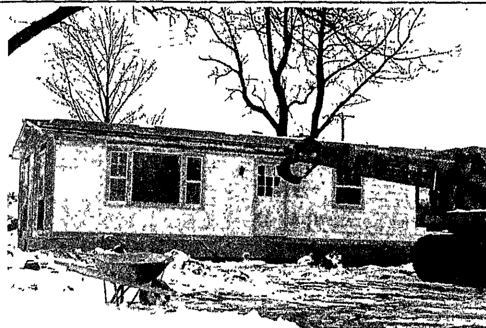
... Both sections in place, only a few details must be attended to before the house is ready for occupancy.
