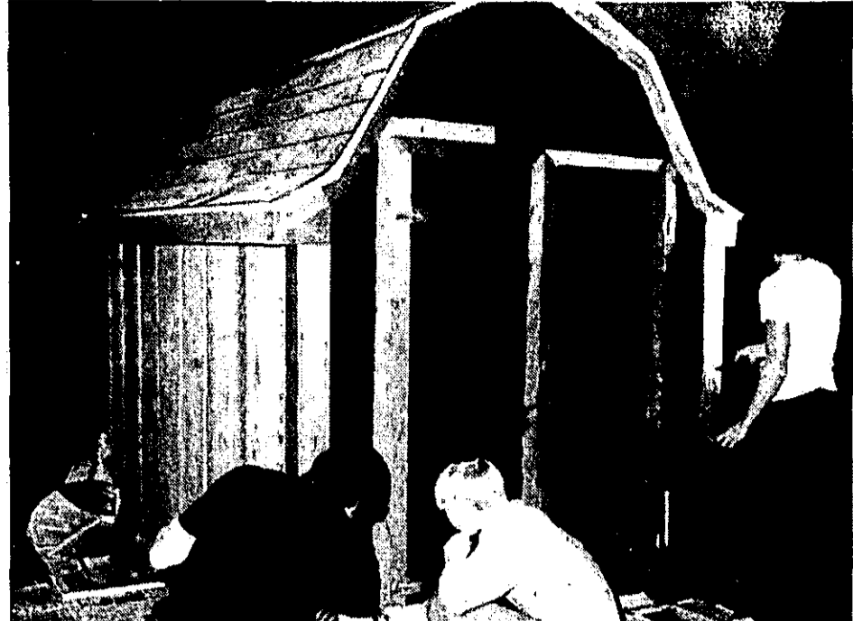
Carpentry classes at St. Johns High School have constructed this storage shed as part of their course work.
