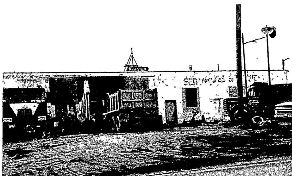
GARAGE TO BE TORN DOWN FOR NEW HOUSING DEVELOPMENT Willard Searles, owner of Searles Excavating, will tear down his garage and office located at 212 S. Scott Road and build a new one on East Walker Road. Searles is well known in the trucking and excavating business. He is presently building a new housing development in this area.
