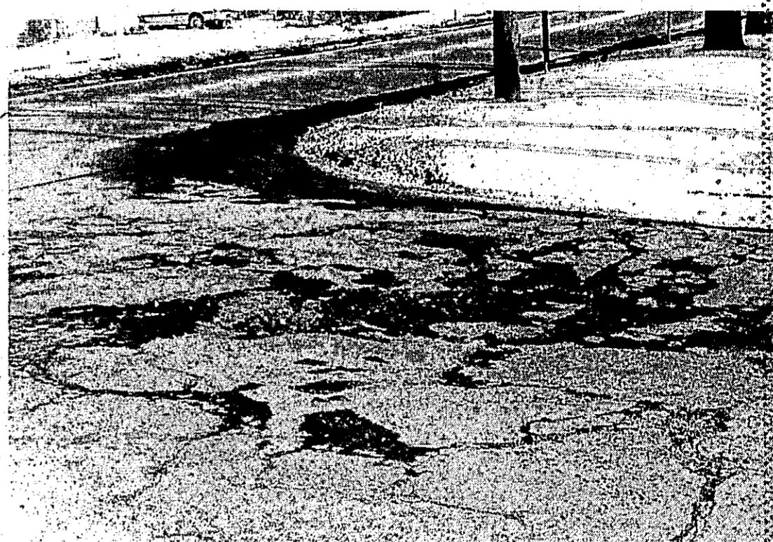
General breakdown of pavement can be seen at the intersection of Lansing and State Sts. The conditions are fairly representative of many areas of the city's street system.
