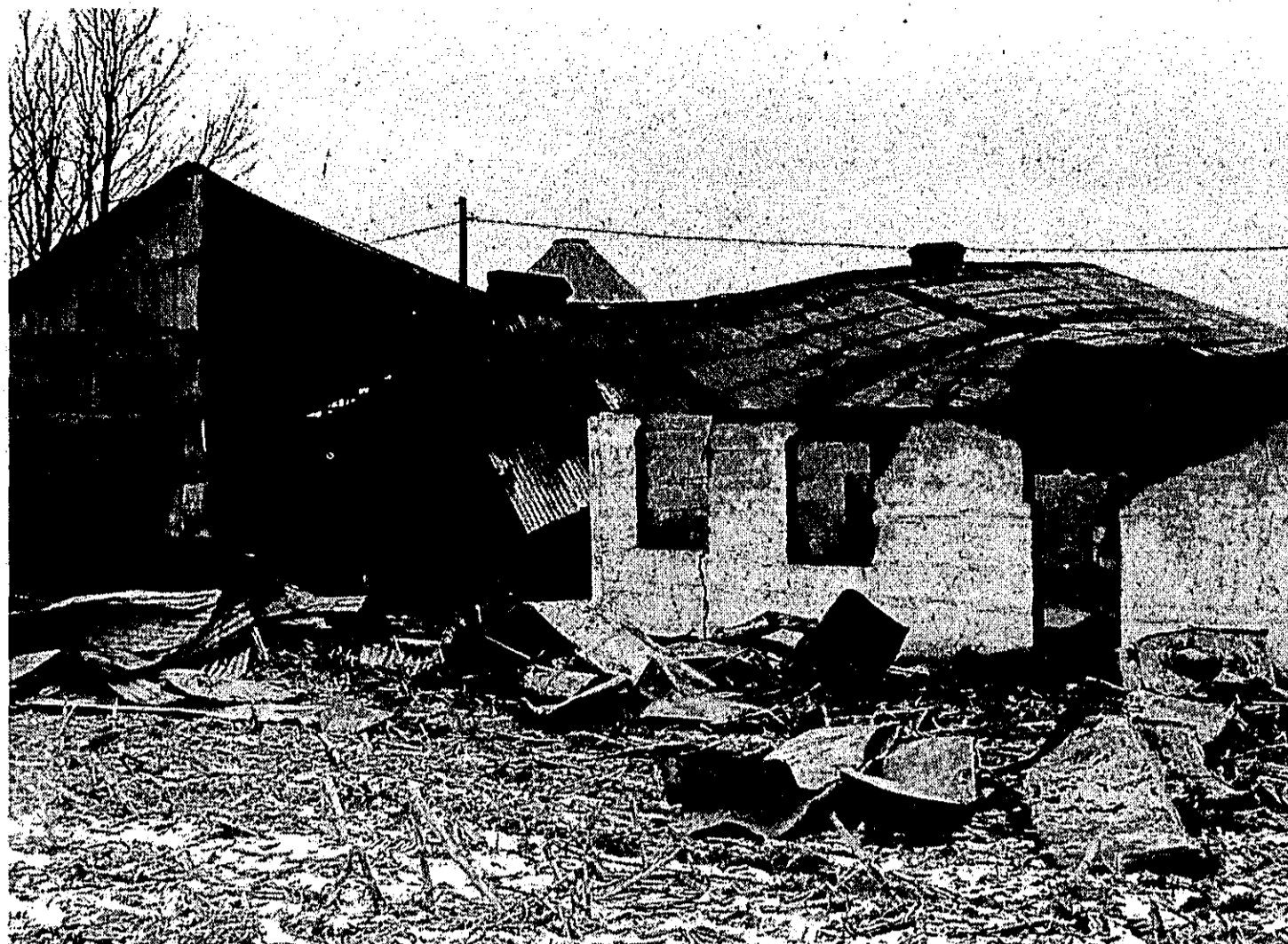
Charred and twisted metal and blackened cement blocks are all that remained of the pole barn and block storage barn on the Robert Wilcox farm south of Shepardsville last Wednesday morning. The buildings burned the evening before, and Wilcox estimated the loss at about $3,500.
