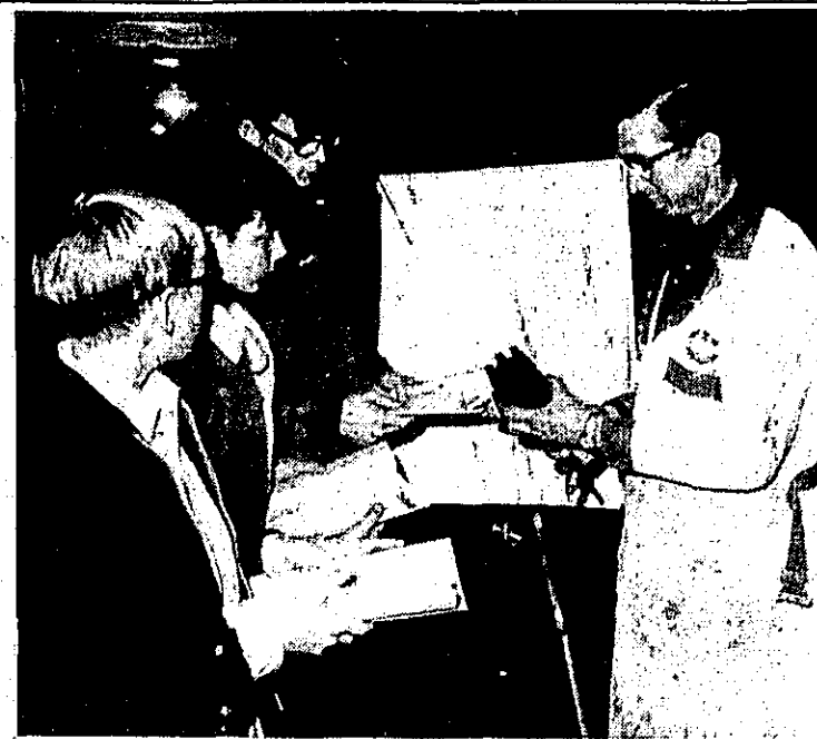
Bernard Feldpausch (right), 4-H automotive leader, explains function of a distributor to Richard Matice of St. Johns, Glen Feldpausch of Fowler and Blaine Stevens of St. Johns.
