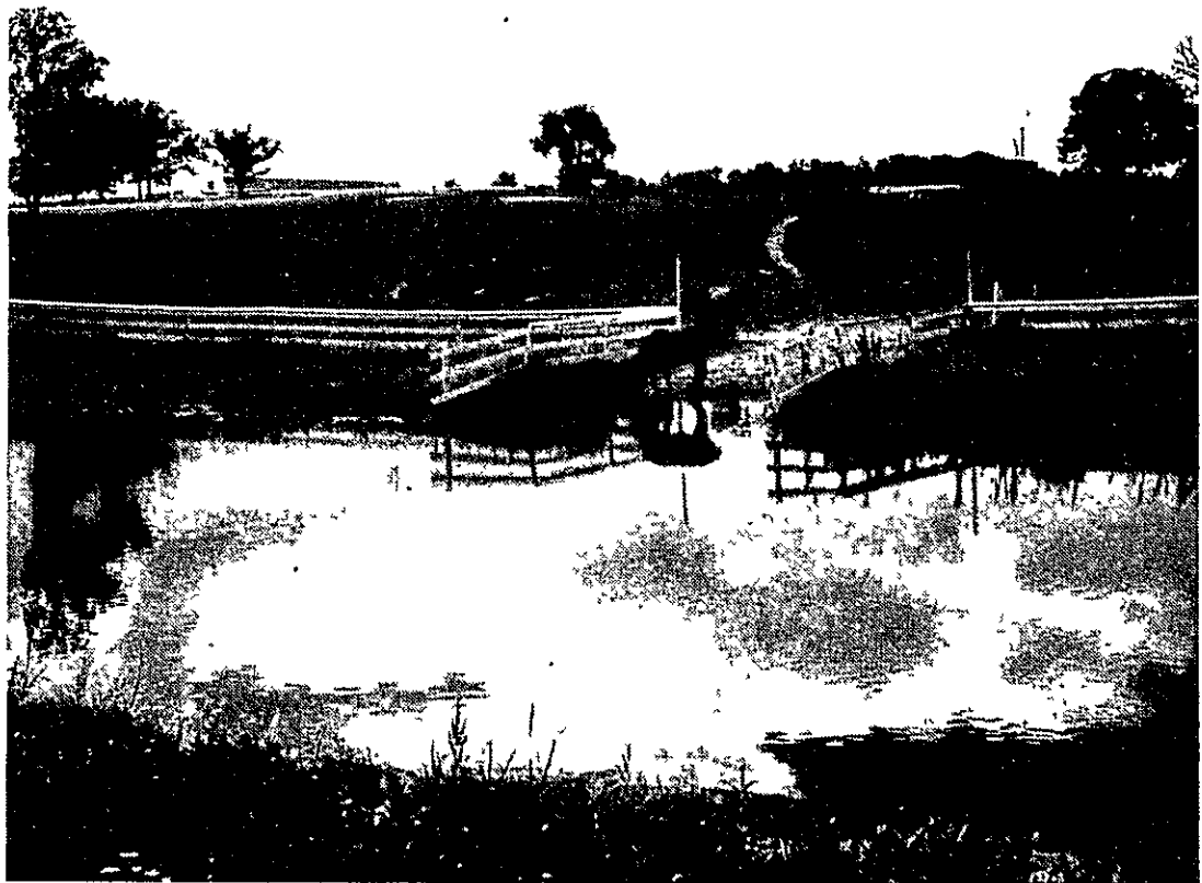
The Livestock pond on the Sidney Bertin Union Stock Farm in Oakland County, Michigan pays off as a source of water for 1 1/2 year old race horses. The pond has two watering ramps which allows watering from separate fields. It was constructed in 1964 as part of a complete soil and water conservation plan developed with the Oakland SCD and provides large trout as an extra dividend.
