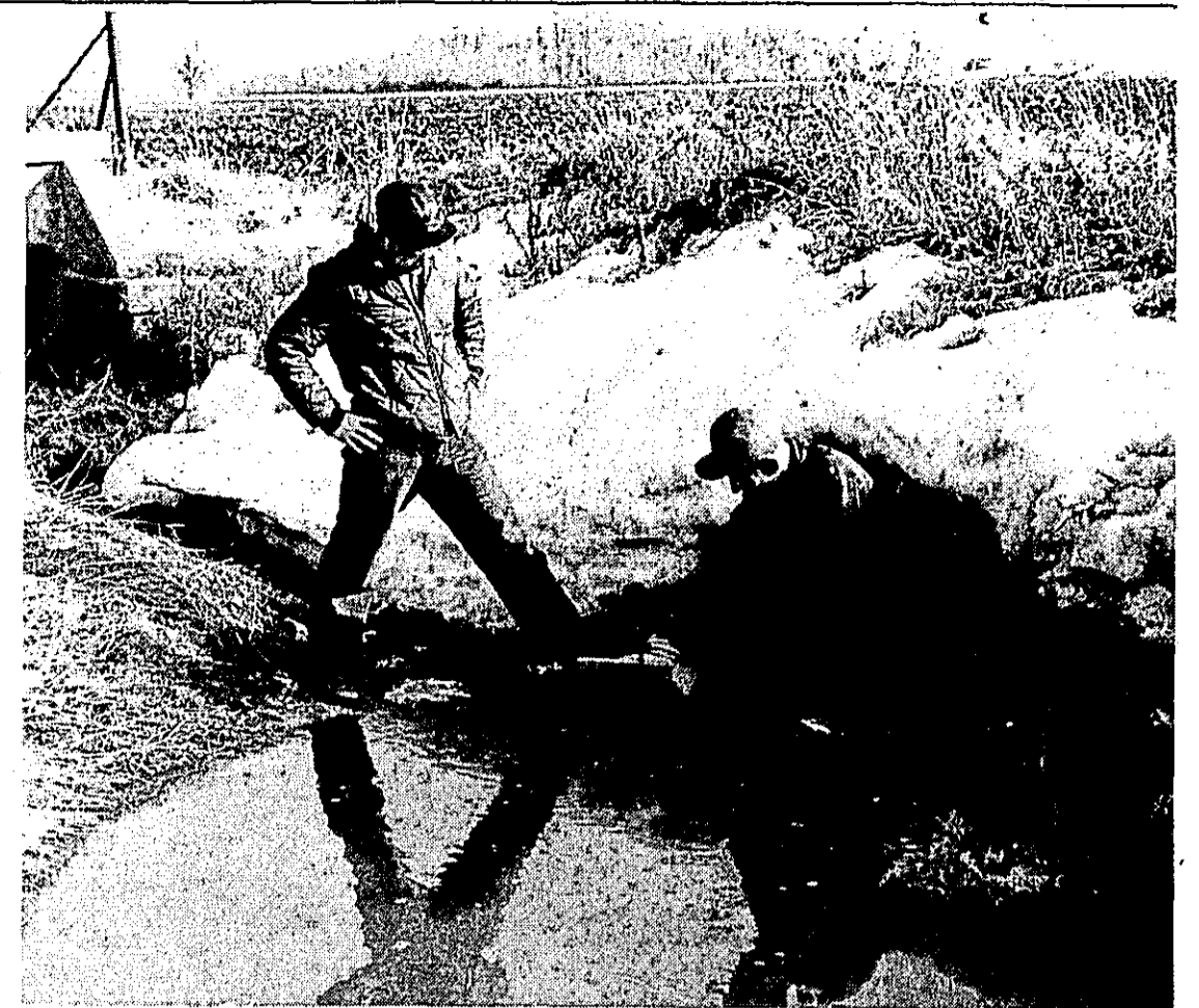
KEEPING TILE MAIN OUTLET OPEN
