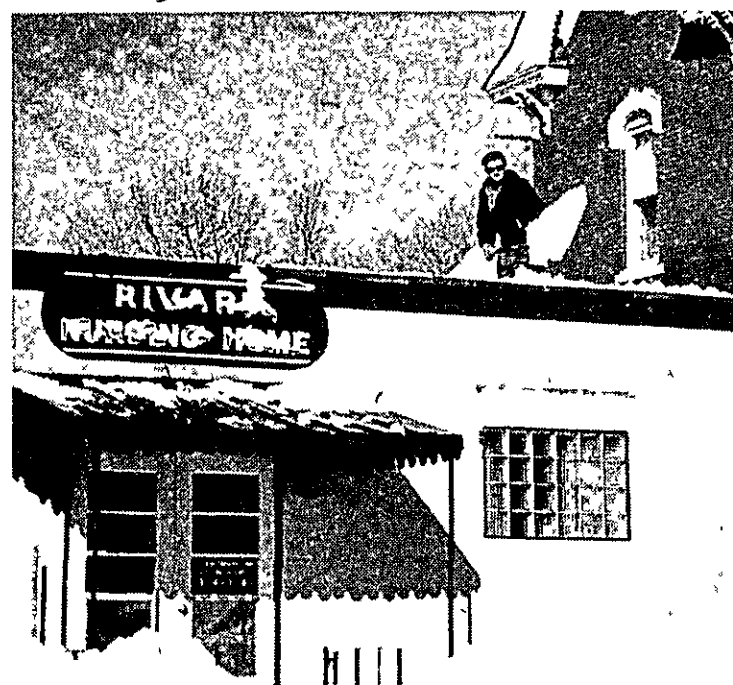
SNOW IS REMOVED FROM ROOF OF NURSING HOME
