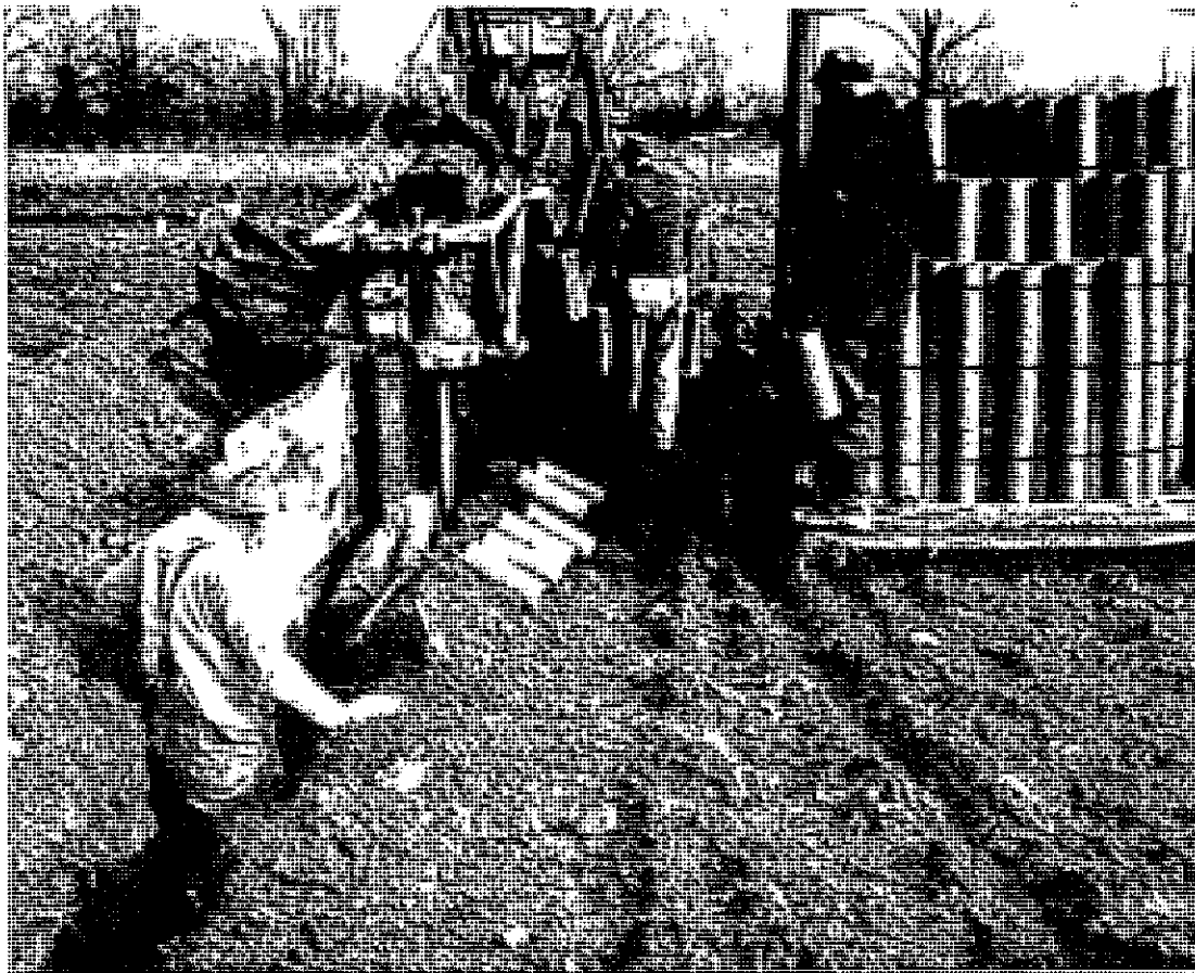
Contractor James Craig installs four-inch tile on the Dale Chapman farm in Lebanon Township. This lateral is part of the planned system for this 40-acre field.
