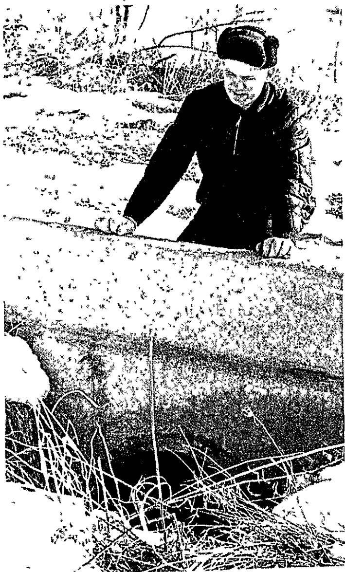
RAY WARNER AND GRADE STRUCTURE
