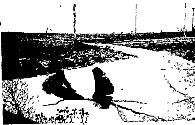
SCS Soil Conservationist Gene Mill and SCS Engineer Frank Cousin examine damaged concrete caused by soil and surface-water problem in the Lansing Mall area. (See Story Page 4)
