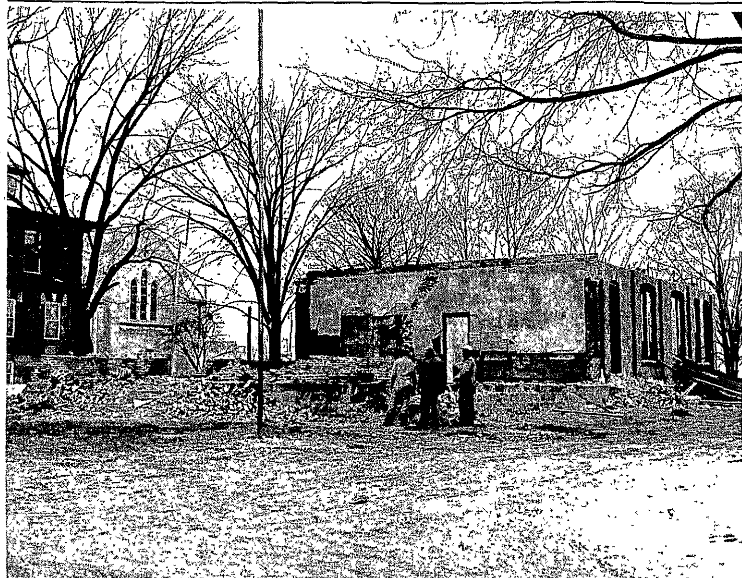
Making Way for New Catholic School at Westphalia
