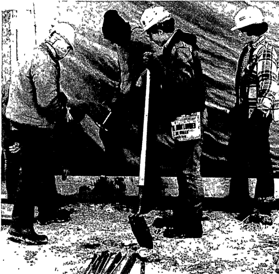
These students ready the garage area so that the floor can be poured accurately.
