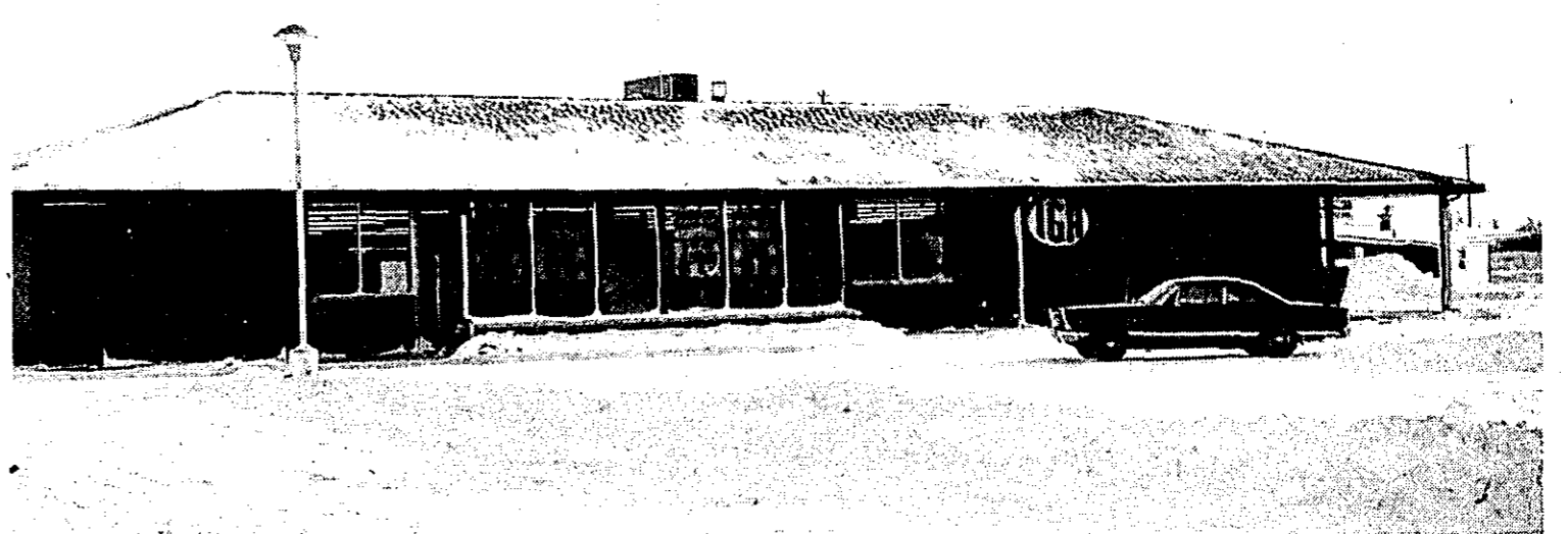
NEW FRONT, ENTRANCE AT ANDY'S IGA
