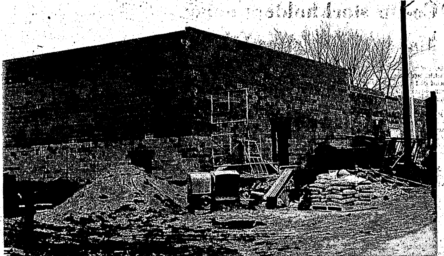
DeWitt Memorial Building Addition Shaping Up
