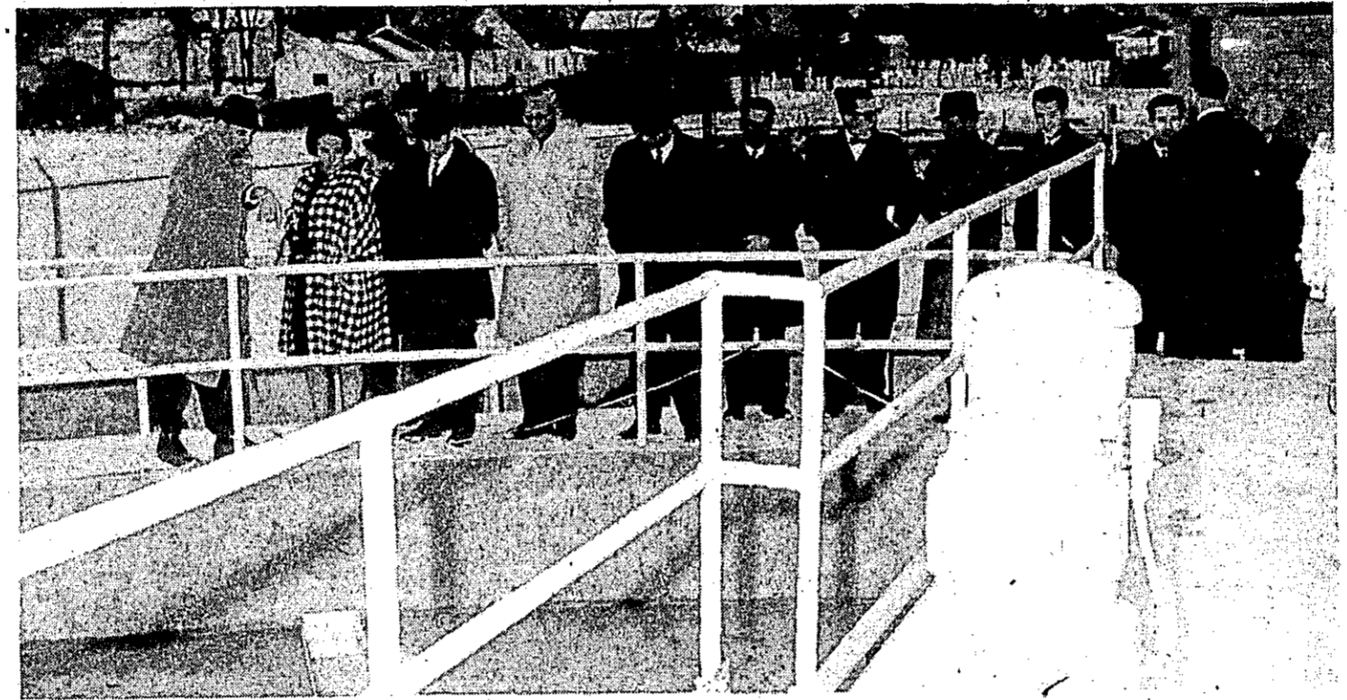
Bob Barnes (left) of Ayres, Lewis, Norris and May explains the operation of the city water plant's clarifier to city officials and invited guests Friday afternoon during an informal dedication program.
