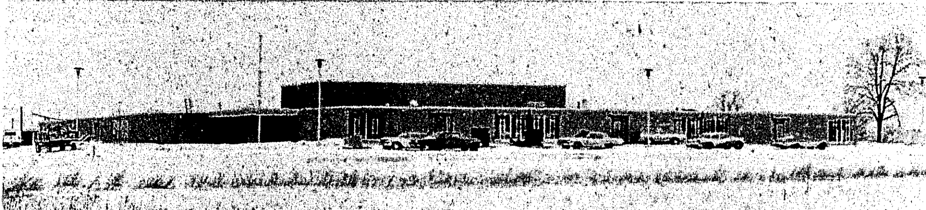
EXTERIOR WORK ALL BUT COMPLETE AT NEW OVID EASTSIDE ELEMENTARY SCHOOL
