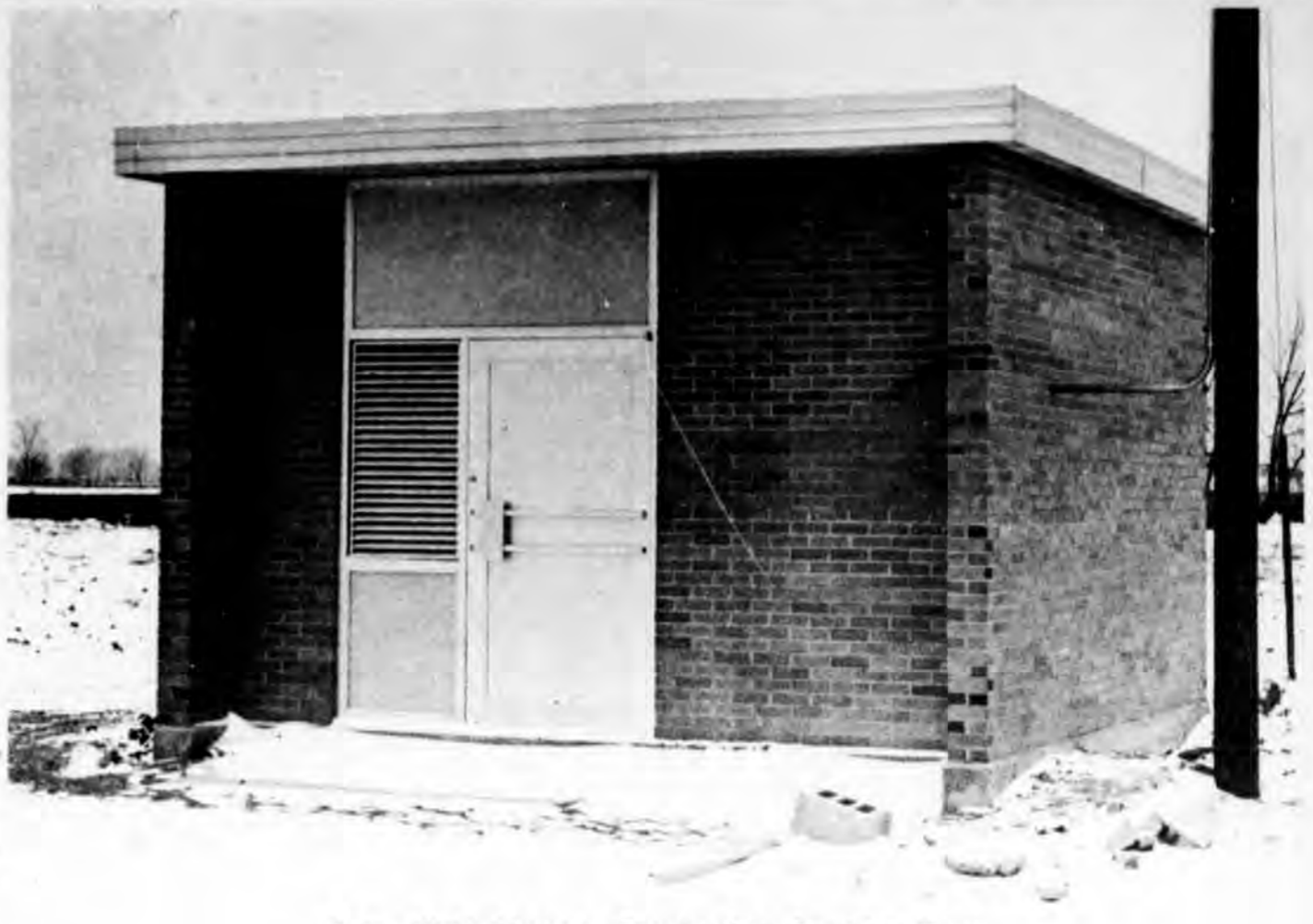
New Well Houses Ready for Standby Duty
