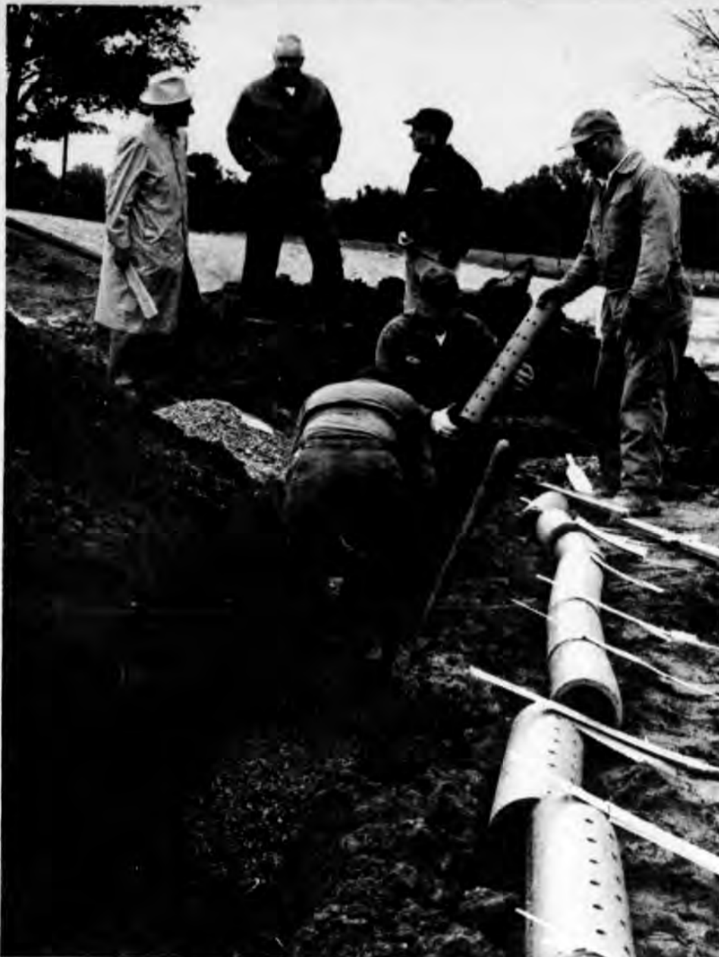
Workmen Put in Field Tile
