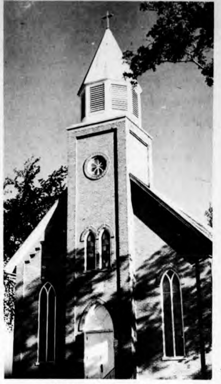
Church Steeple Finished
