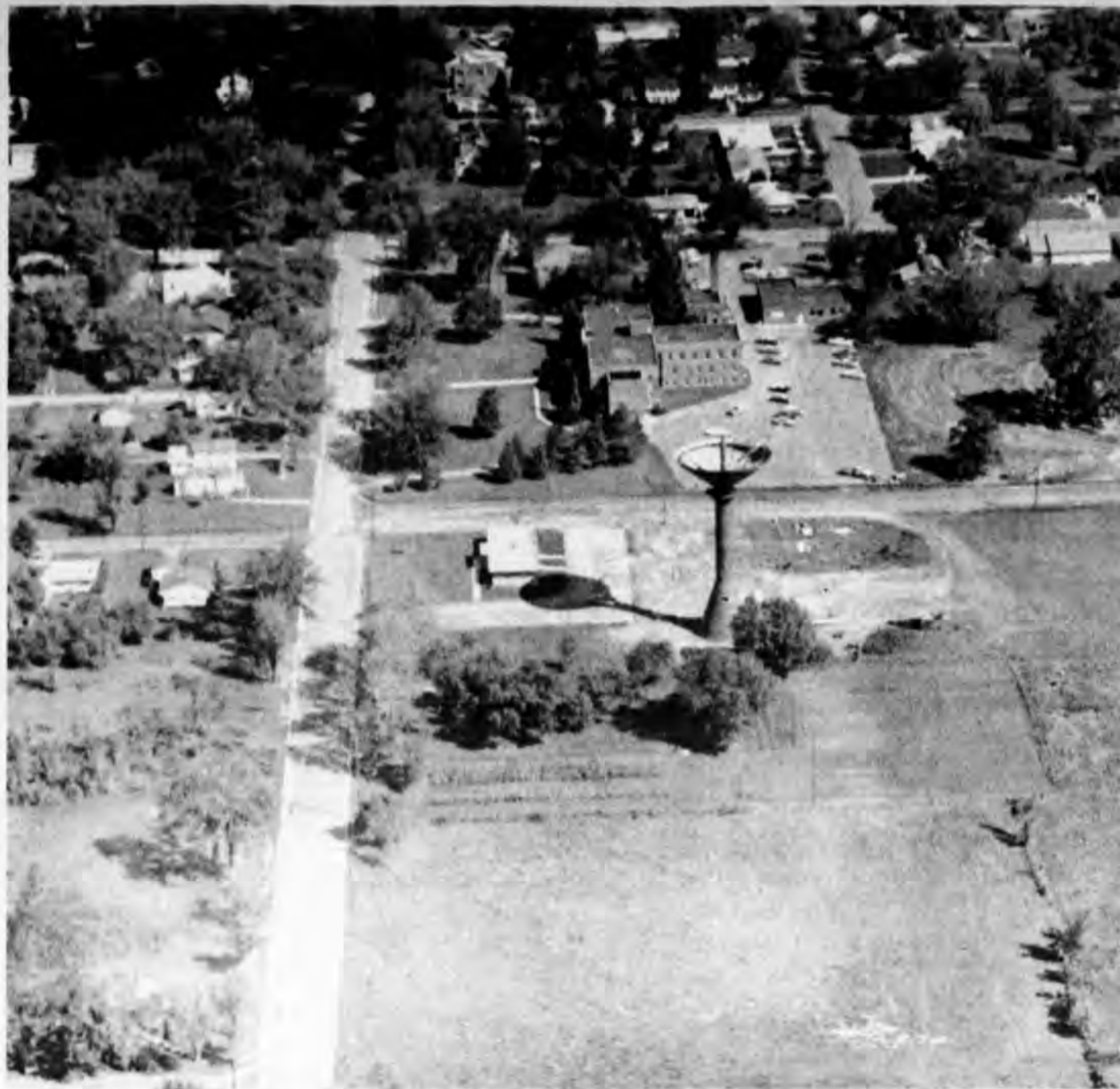
New Water Tower Imposing Sight on City's South Limits
