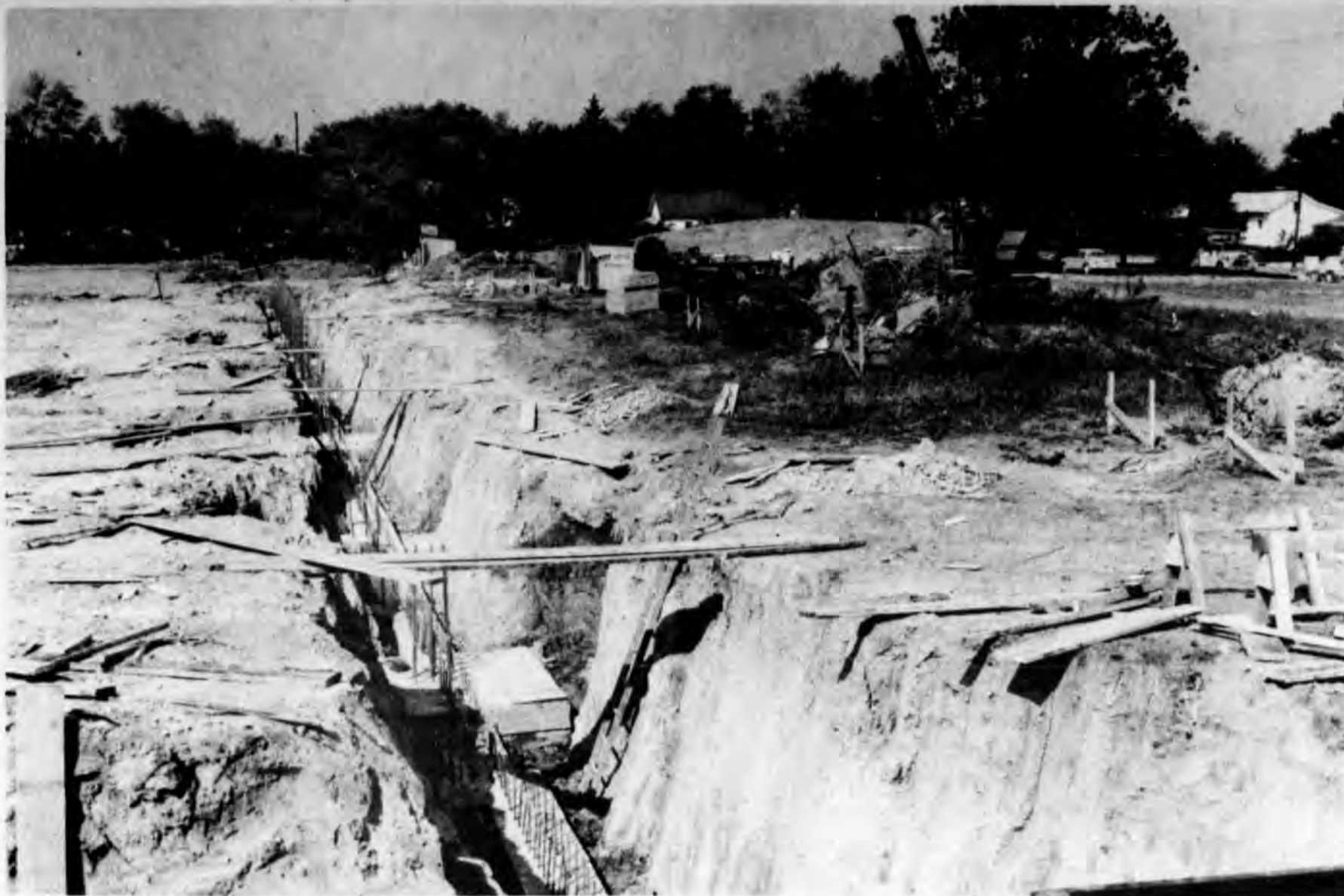
Expanse of $3 Million Federal-Mogul Addition Shown By Excavations
