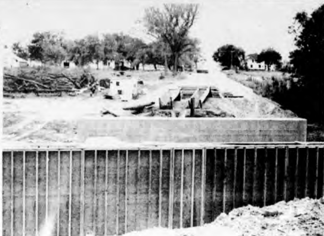
Supports for New Wood Road Bridge
