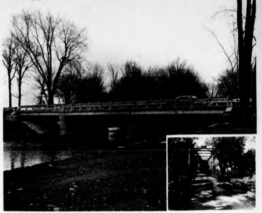
On Upton Road Crossing Looking Glass River View of old bridge (inset lower right)
