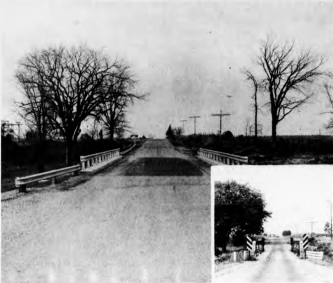
On Forest Hill Road Crossing Hayworth Creek View of old bridge (inset lower right)
