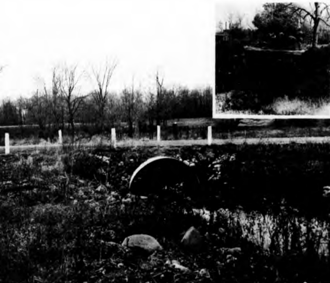
On Clark Road at Niles Road View of old bridge (inset upper right)
