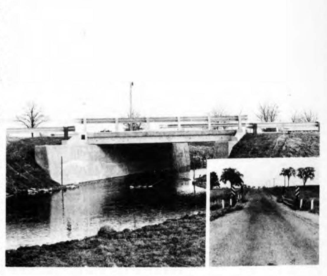
On Forest Hill Road Crossing Cox Drain View of old bridge (inset lower right)
