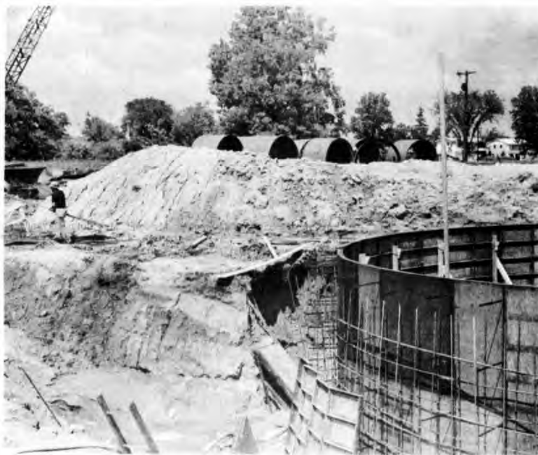
Workmen are in the final stages of construction of the base for the new water tower south of the hospital. Framework was nearly complete last week prior to pouring concrete. Visible in the background is steel which will be used later.
