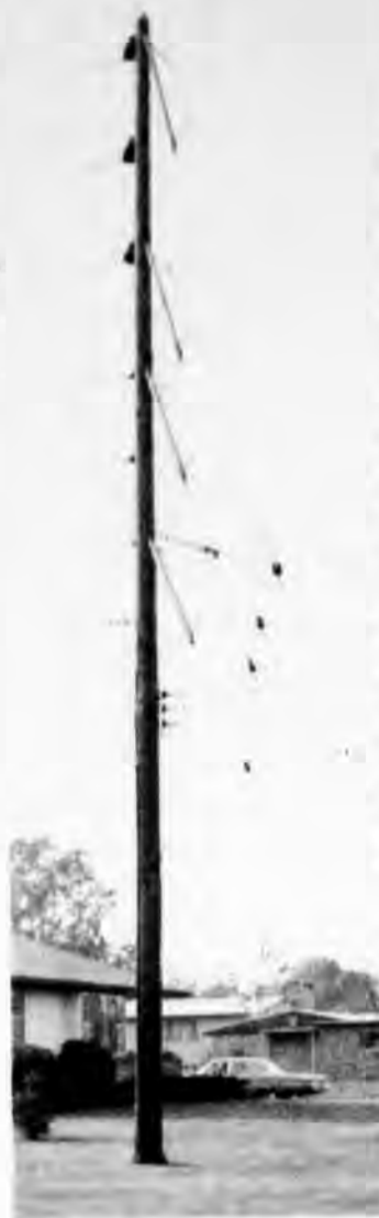
Poles like this rigged on square corners of power line routes are one of the things folks near the corner of Sturgis and Swegles streets are protesting.
