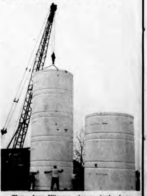
These Aqua-Nitrogen storage tanks have a capacity of 22,000 and 11,000 gallons.
