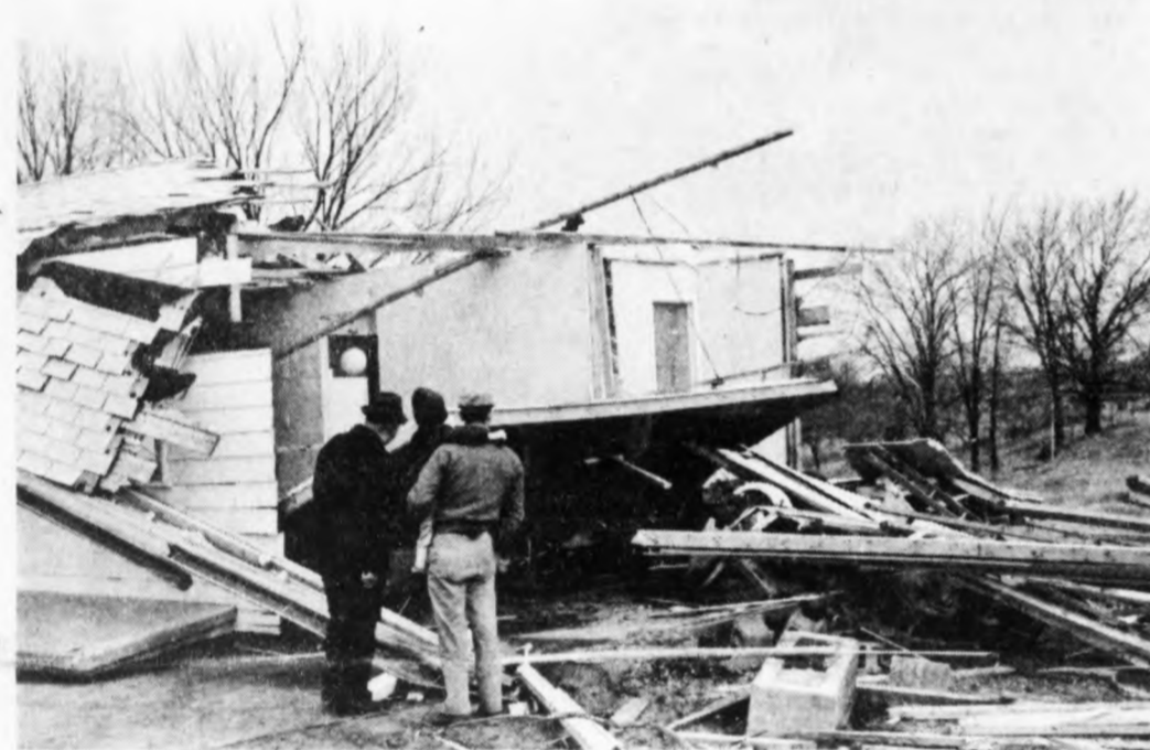
A tornado which hit south of DeWitt on Palm Sunday evening killed one girl and injured four others, demolishing this and four other homes.
