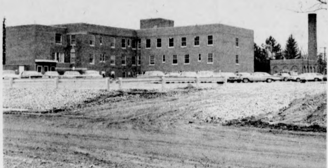
New Parking Entrance at Clinton Memorial
