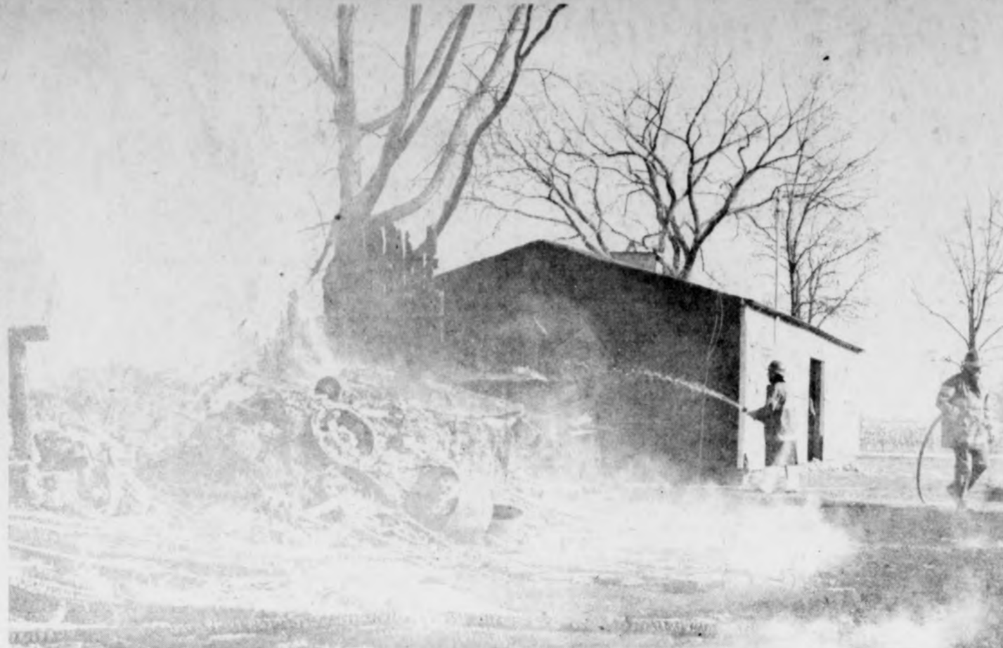
Tool Shed, Grainery Near Maple Rapids Leveled by Fire
