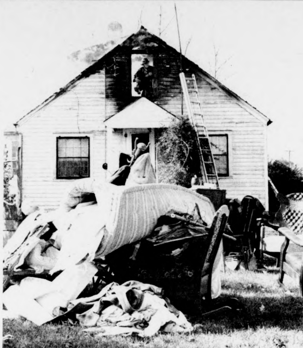
Fire Damages Coykendall Home
