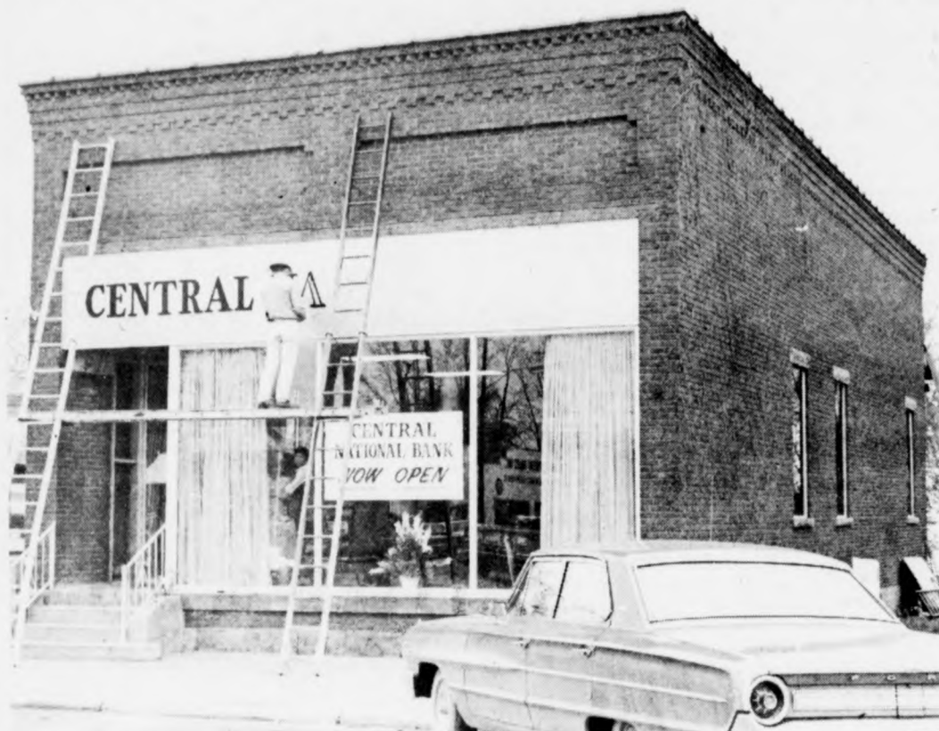
The finishing touches are put on the outdoor sign at the Central National Bank's new Pewamo branch office last Thursday when the bank opened its doors for business. The remodeled interior of the old bank building is paneled and carpeted.
