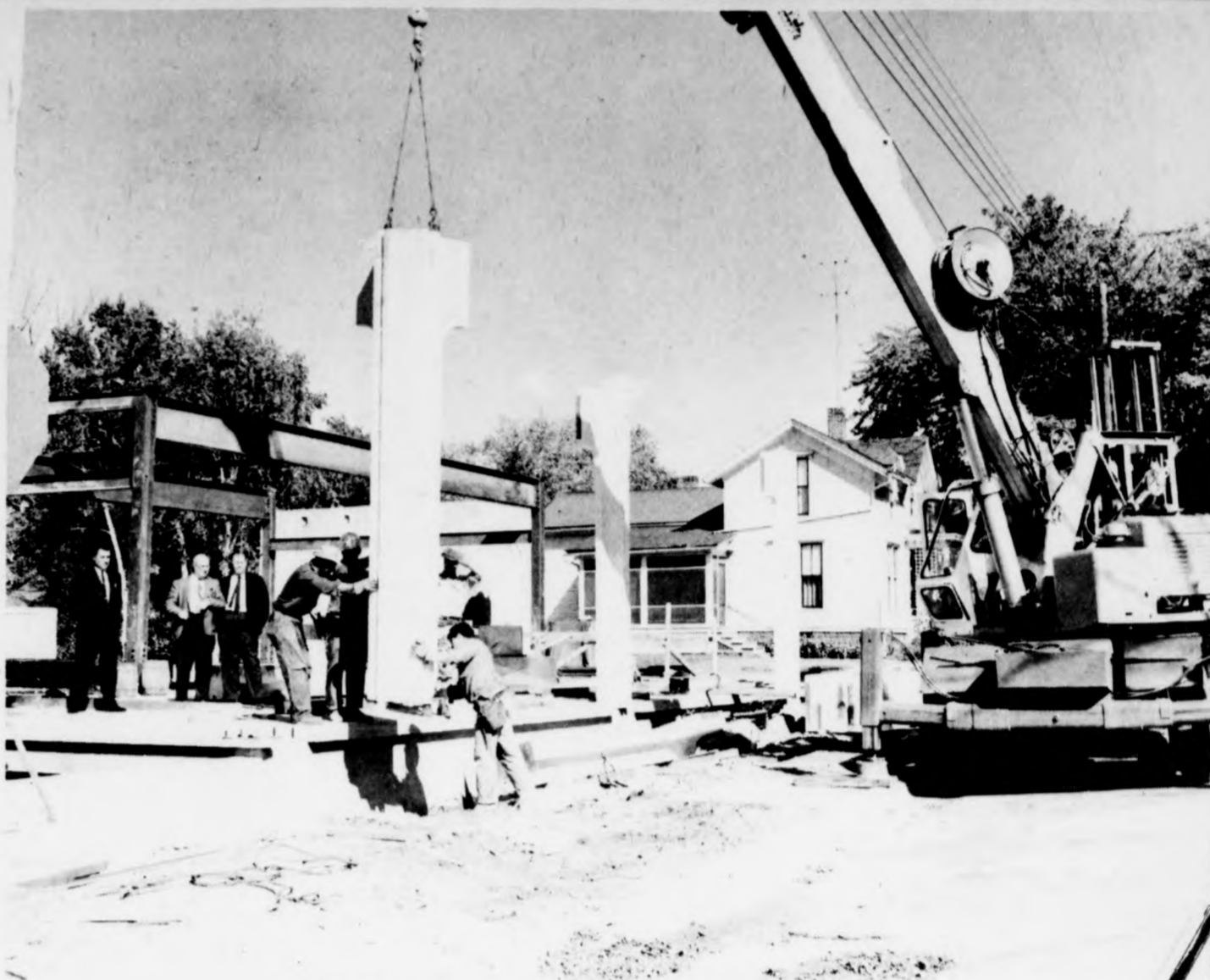
Pillars for New Bank are Swung into Place
