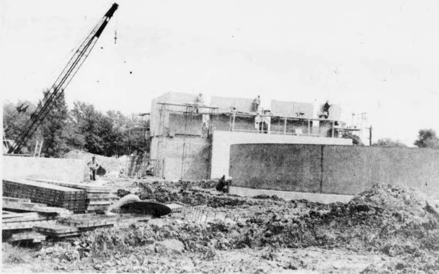
Looks Like Major Project at Water Treatment Plant
