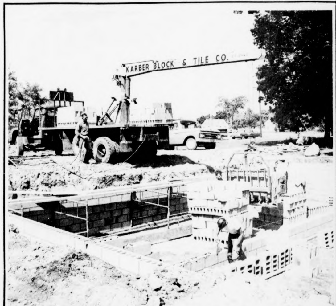
Kaufman Construction Co. takes full advantage of Karber's Side-O-Matic Delivery. Pictured above is a load of blocks being lowered into the basement of a new home being constructed in Elsie by the Kaufman Construction Co.
