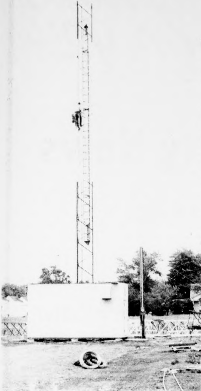
Workers High Up in the Air
