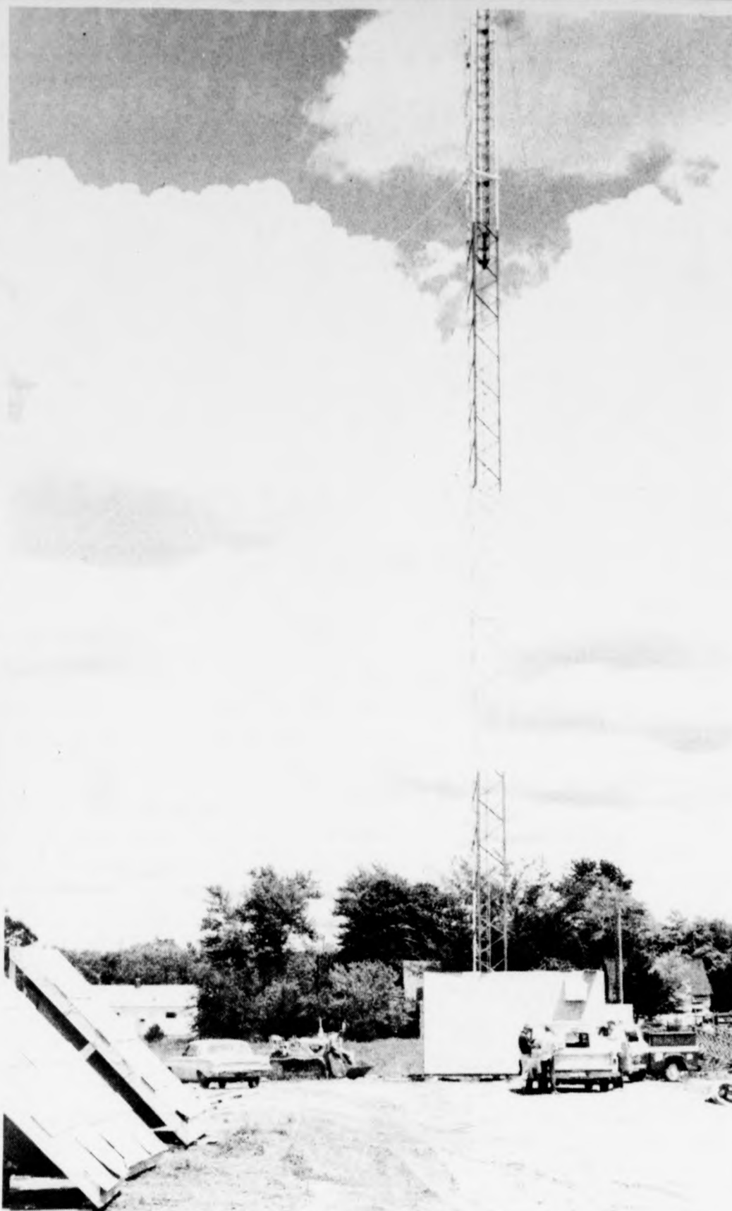
Reaching for the clouds now, this lower section of the new General Telephone Co. microwave tower at the west edge of St. Johns is only about 40 percent of its completed height at the stage shown here. The tower at this point is 125 feet; when finished it will be 305 feet. Antennae for the tower are in the crated containers at left. This view looks east toward Morton Street.
