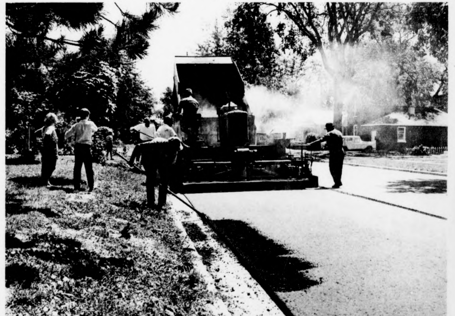
Asphalt Replaces Gravel on Two Blocks of West Sturgis Street
