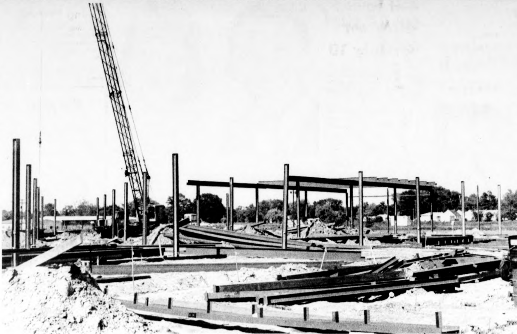
Patterns in Steel Begin to Form at Sealed Power's Plant
