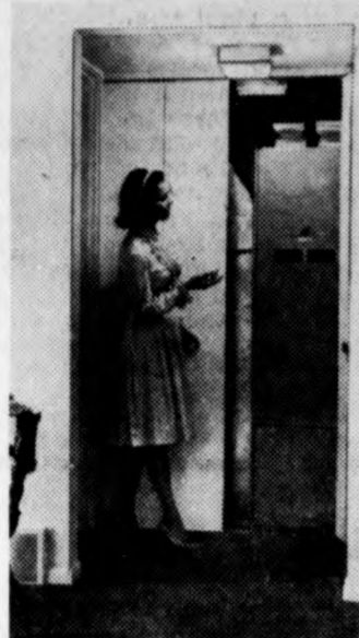
HIDDEN IN a closet is electric furnace which can heat an entire home. It can also be combined with central air conditioning. By American Furnace Co.
