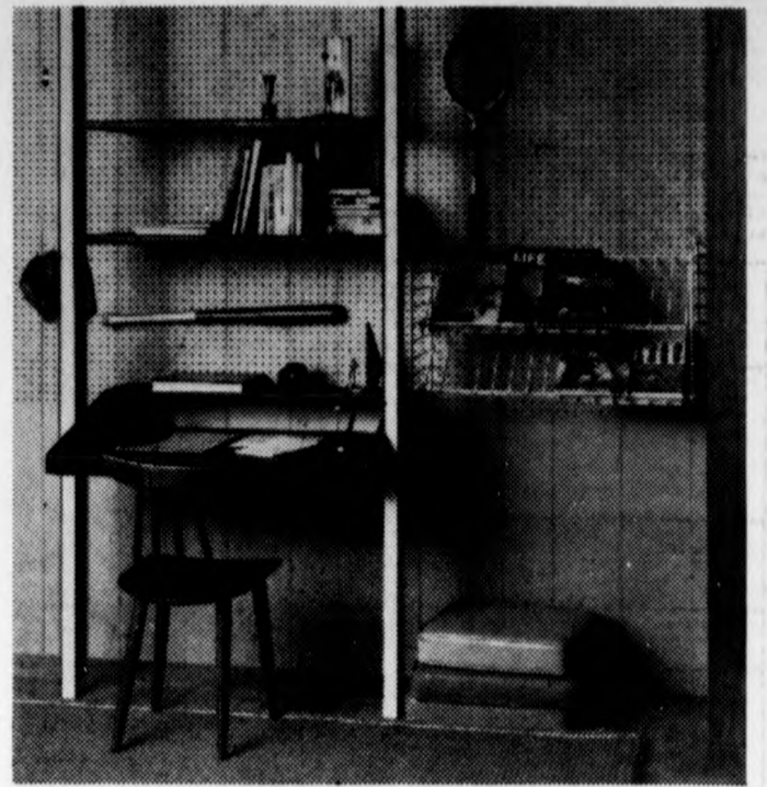
FROM THE GARAGE TO THE STUDENT'S corner goes this factory-finished hardboard. Originally designed as a garage liner, paneling has lower three feet fashioned as a solid wainscot, with top perforated to act as storage wall for books, souvenirs.
