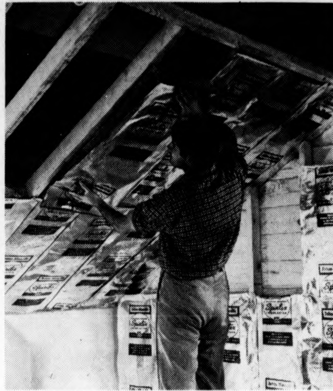
PROPER INSULATION DOES MUCH TO cut heating and cooling costs, since it holds in the heat in winter and does the reverse in summer. In accessible area, such as the attic, the homeowner can easily install insulation himself. Insulation here by Johns-Manville.
