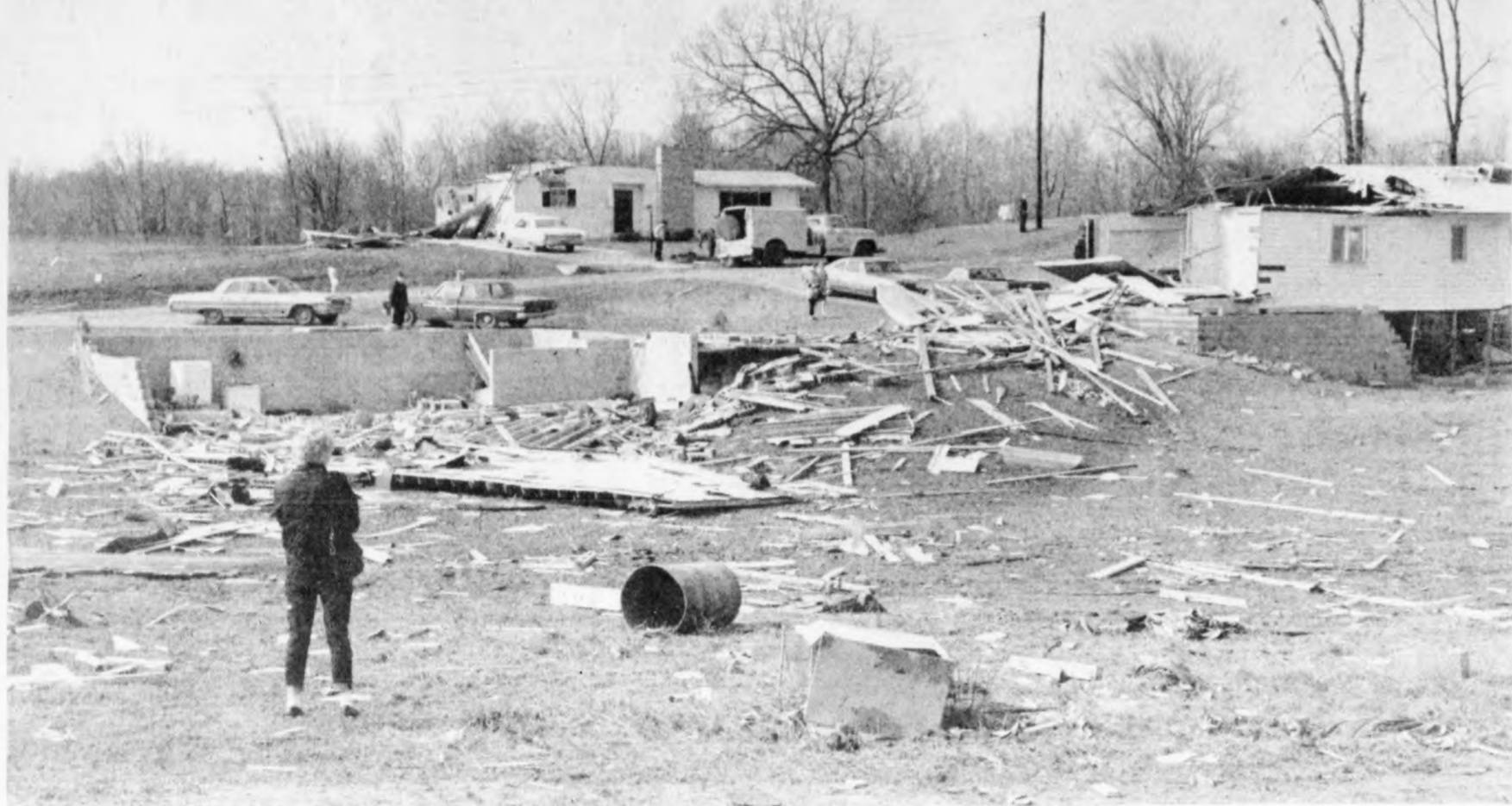
A woman surveys all that's left of three homes on Theresa Street in DeWitt Township after Sunday evening's tornado smashed them down. Only the foundation remains of the William Eckerle home (nearest the woman). Directly behind it on the hill
