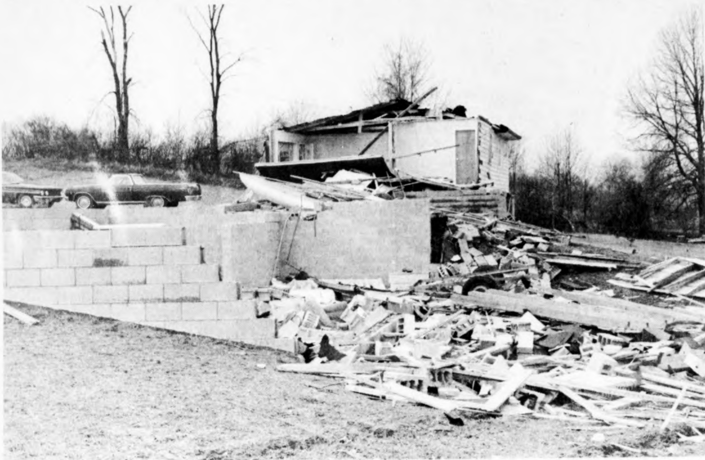
Only Concrete Blocks Remain of Home Where Child Died in Tornado
