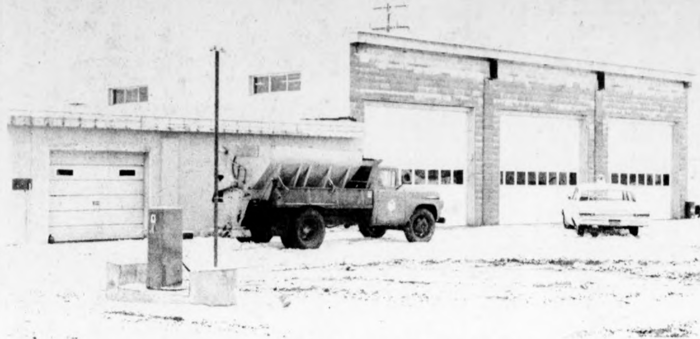
New City DPW Building on North US-27
