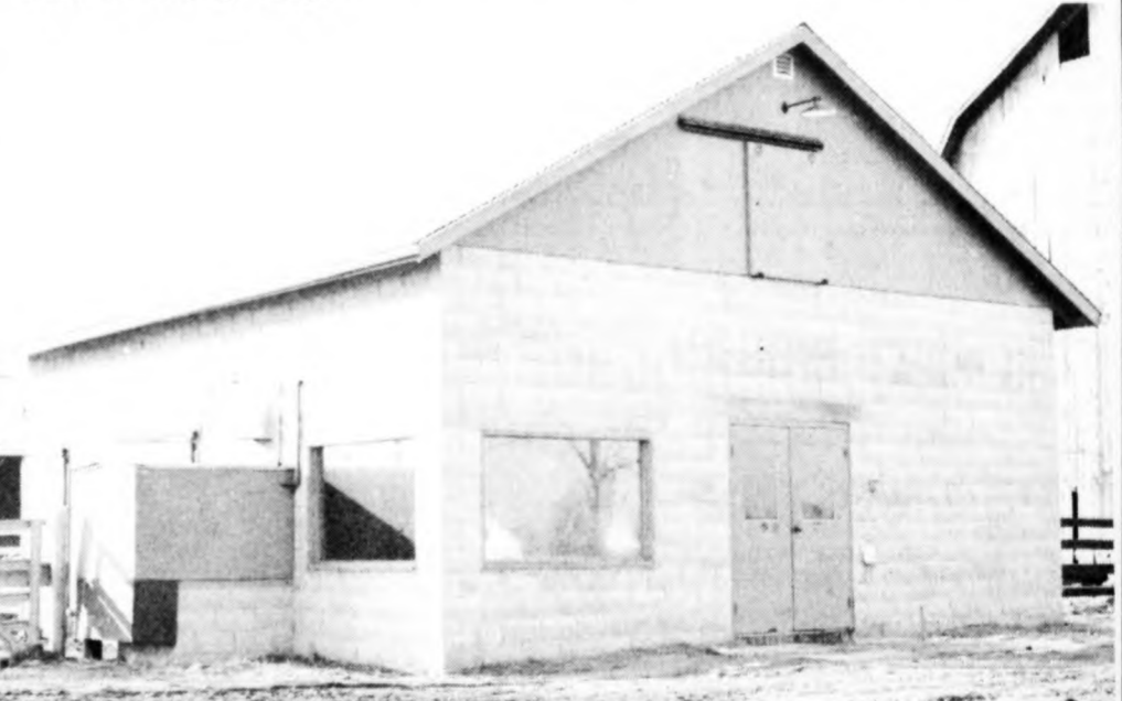
Shown above is the 28x32 milking parlor owned by Raymond D. Thornton, Duplain township dairyman. The milking parlor was constructed with Karber's Insulated Blocks.
