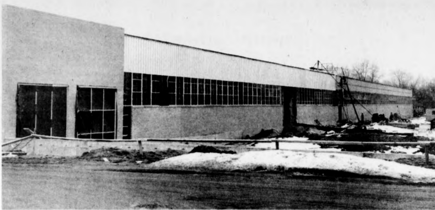
Federal-Mogul Plant Has Imposing New Look from North Mead Street
