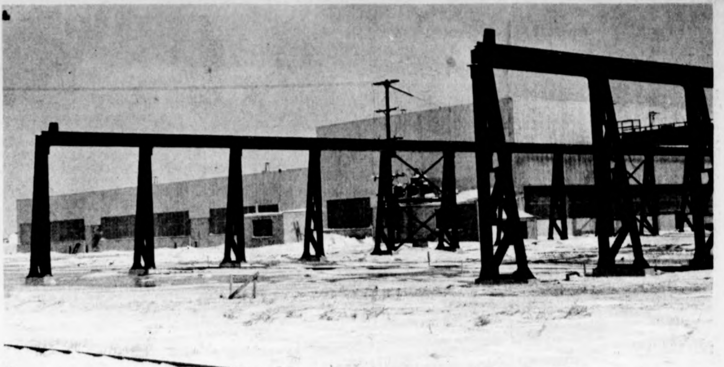
This exterior view of the new Ashley Corp. plant shows the dark steel overhead tracks that will be used by a big crane to move steel. Main Ann Arbor Railroad track is at lower left of the picture, and a railroad siding goes between the second and third crane-track supports.
