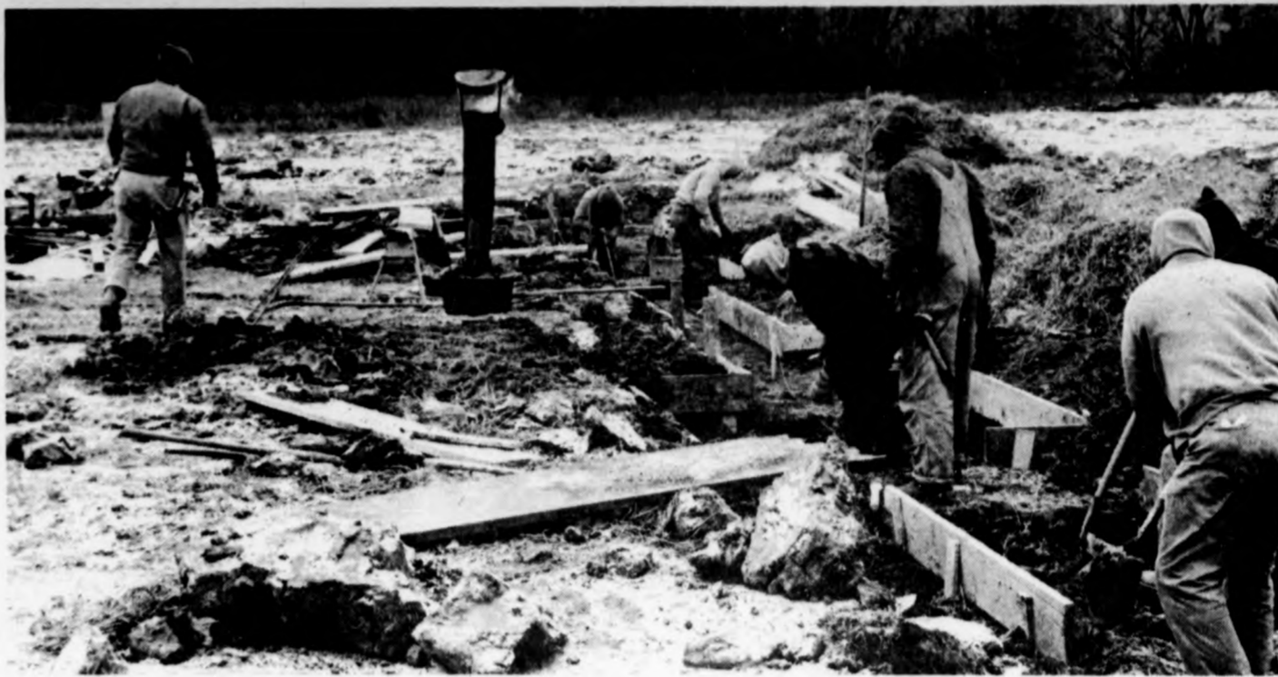
Workmen Brave Cold on DeWitt High School Job
