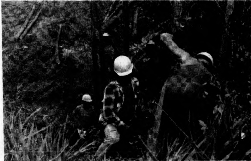
Crews clear brush
