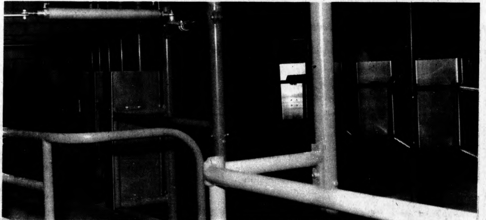
New York visitors admire the milking parlor under construction at the Nobis Farms. Walls are a soft blue color on a smooth glazed surface that would look attractive in a home, yet alone a barn.
