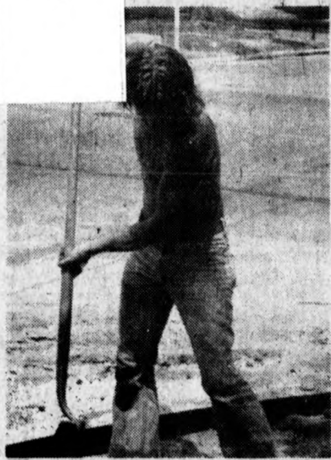
Kurt Woodbury levels cement
