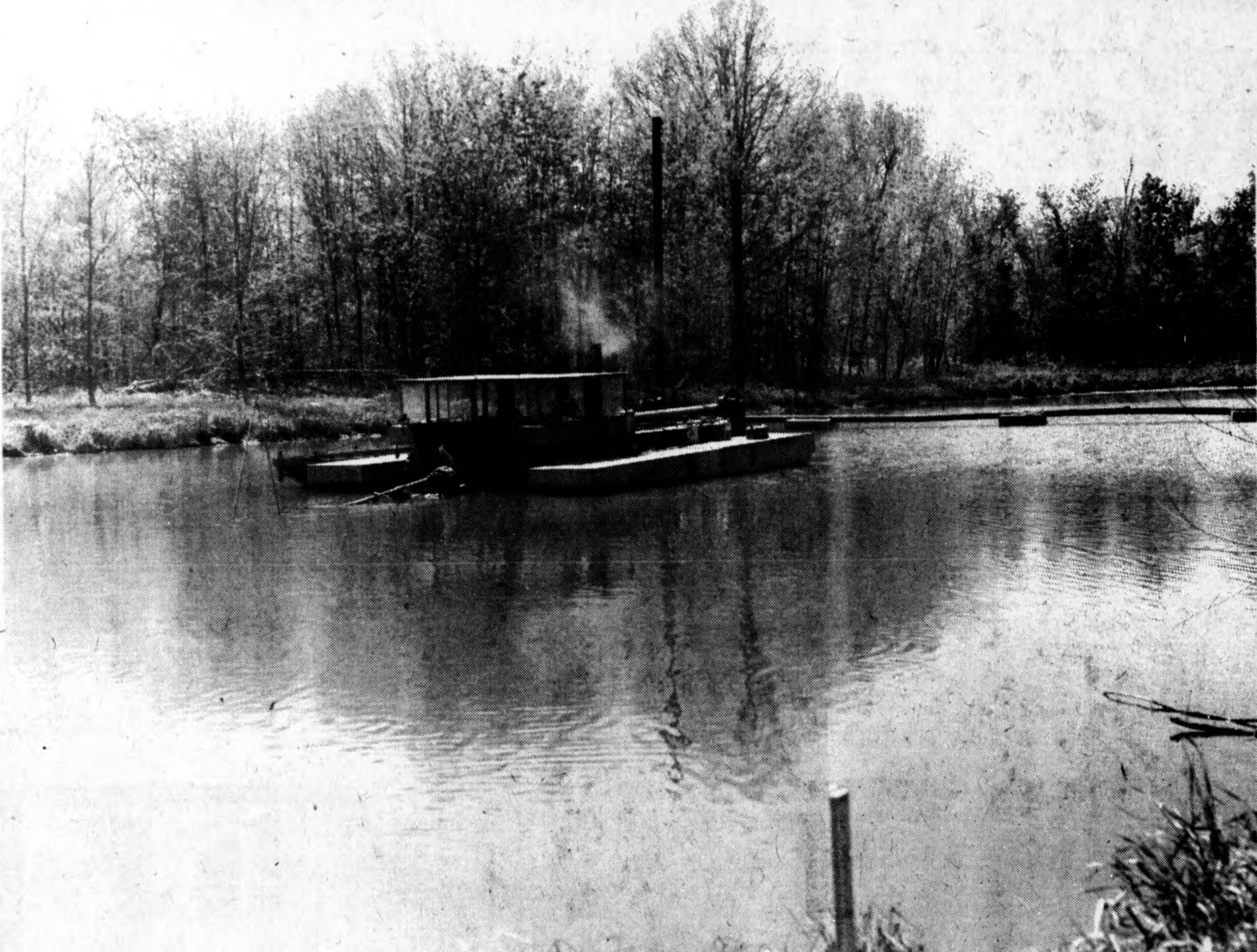
Suction dredge removes sediment from Maple River
