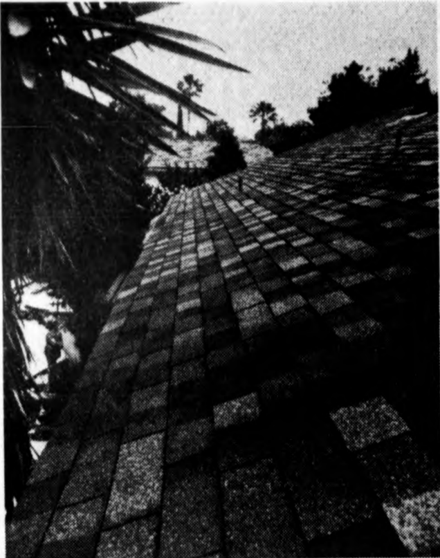
FIBER GLASS SHINGLES from Johns-Manville look just like conventional shingles, but last longer and will not swell or shrink in humid weather. And, while most traditional shingles are U.L. listed Class C for fire-resistance, fiber glass shingles are given top rating — Class A. The benefit to homeowners is the best fire protection available.
