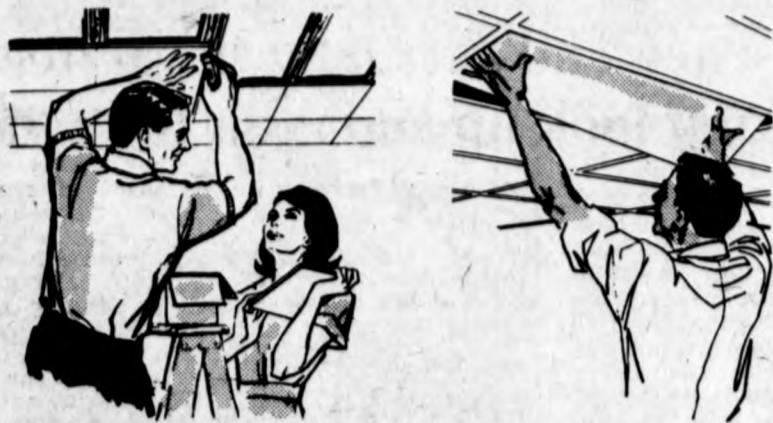
FOR NEW CEILINGS, Johns-Manville says tiles are normally 12 inches square and applied to furring strips over existing ceiling (left). Lay-in panels are 2-ft. by 4-ft. and drop into a suspended grid system of metal supports (right).
