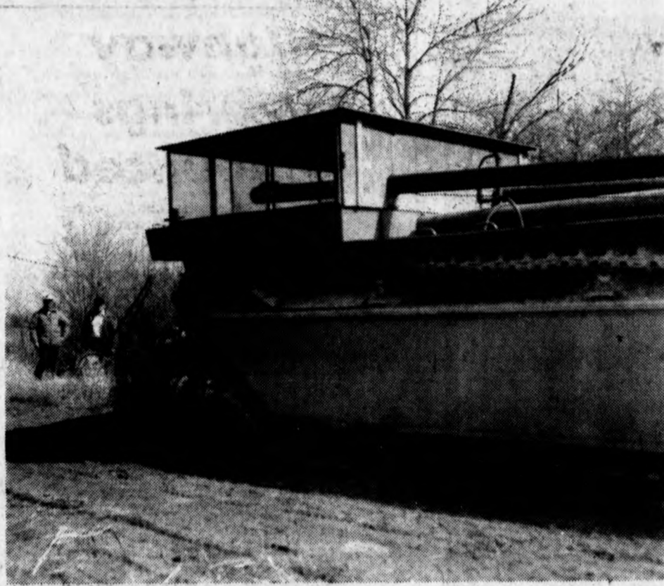
William P. Repp (left), government inspector; and Jack W. Elder, project engineer, Soil Conservation Service, Watershed Construction Unit, inspect the 8-inch suction dredge that will be used on the Maple River.
