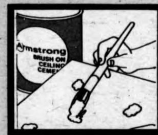
CEMENT directly onto sound existing ceiling...
