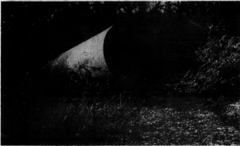
The Steel-Wallbridge Drain, south of St. Johns, protrudes up and out of the drainage area. City and county engineers termed the drain useless. The County Drain Commission will now reinstall the tube and redirect the flow of water to make the area functional again. (Photo by Marty Ackley)
