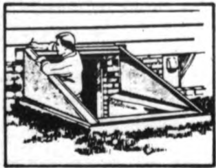
Assemble frame and fit to house.
